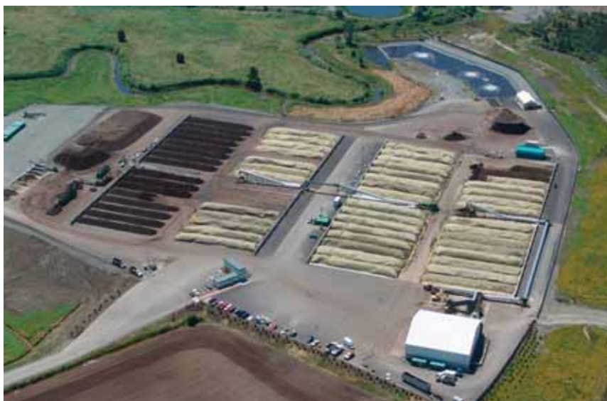
THE COMPOSTING PLANT IN EVERETT, USA. IN THE COMPOSTING PLANT IN EVERETT, USA THE GORE™ COVER SYSTEM HAS SUCCESSFULLY BEEN IN OPERATION SINCE 2005, TREATING ORGANIC WASTE AND GREEN WASTE AND ACHIEVING A THROUGHPUT OF 160,000 TONNES PER ANNUM.
